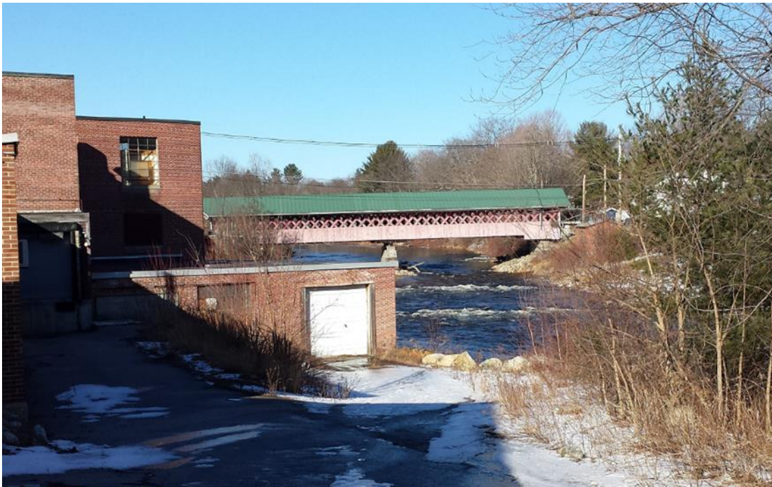
Homestead Woolen Mills Dam and Thompson Covered Bridge Over Ashuelot River
